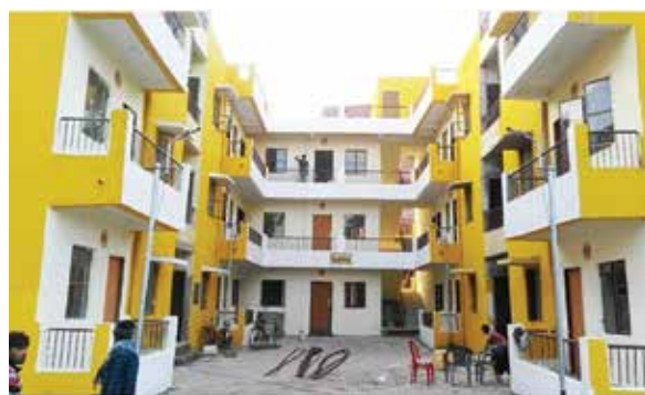
Demonstration Housing Project using Coffer Structural Stay in Place Formwork System at Biharsharif, Bihar
