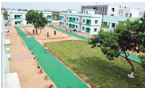
Demonstration Housing Project using Glass Fibre Reinforced Gypsum Panel System at Nellore, Andhra Pradesh
