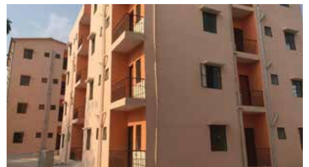
Demonstration Housing Project using Coffer Structural Stay in Place Formwork System (16 houses) and Light Gauge Steel Frame System (16 houses) at Gachibowli, Hyderabad, Telangana
